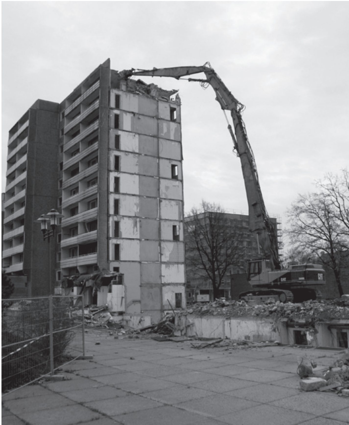
Demolition of a building in Cottbus, Germany. Photo: Stefan Schroeter
