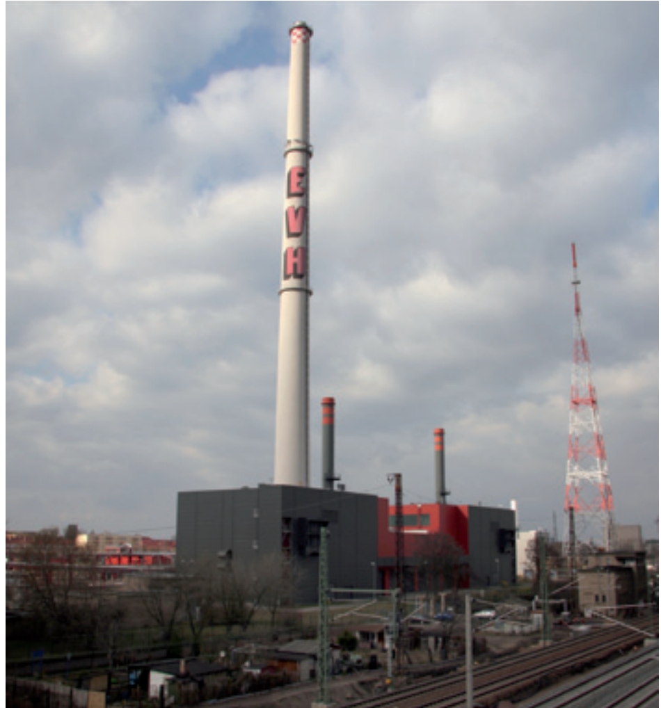
With its two cogeneration installations, the new Dieselstrasse heat and power station can respond flexibly to heat demand in winter and summer. Photo: Stefan Schroeter
